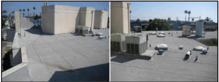
The roof appeared generally serviceable.
