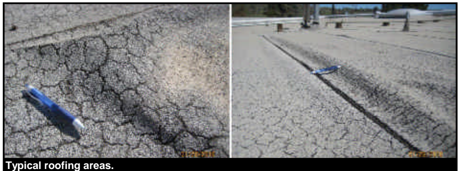
Typical roofing areas.
