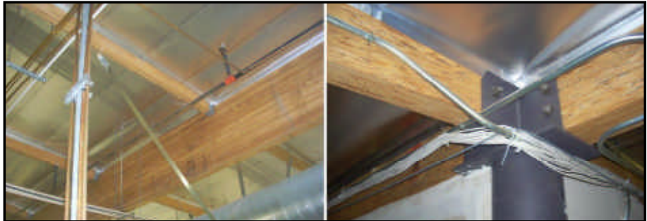
View of beams and cross supports
