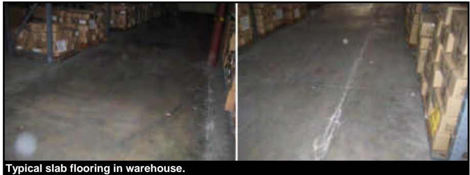
Typical slab flooring in warehouse.
