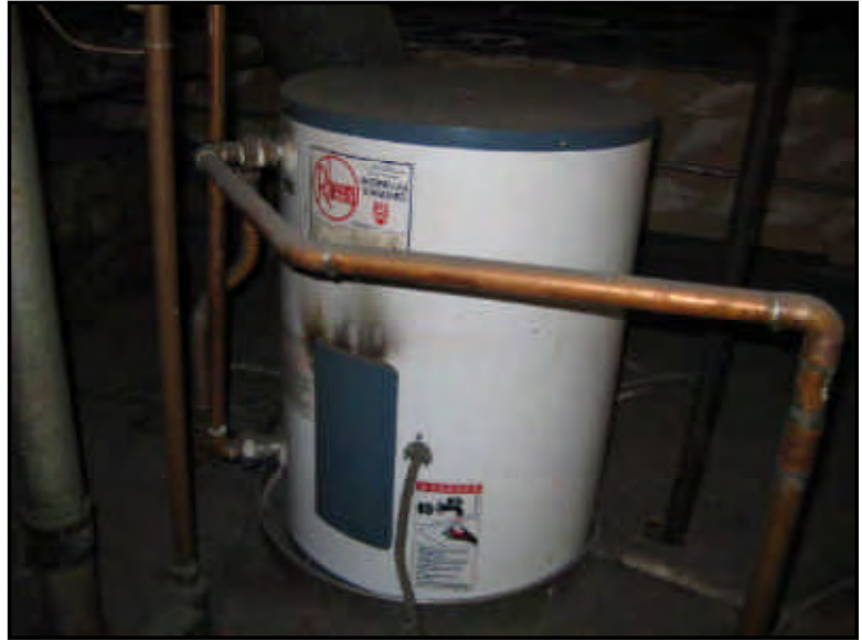
Over the bathroom near the roof access ladder.
