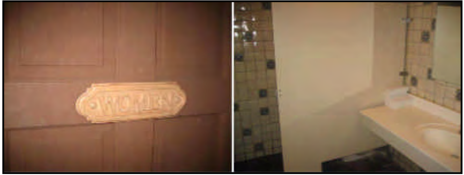
Womens Restroom upstairs
