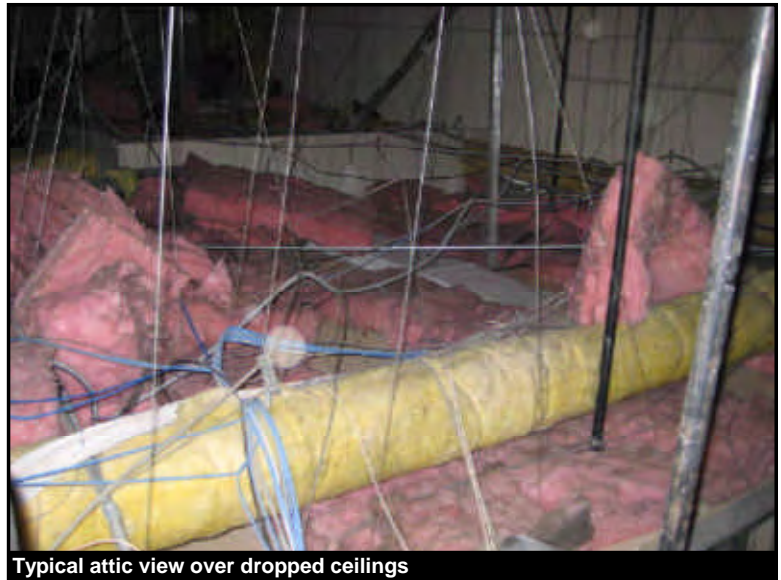
Typical attic view over dropped ceilings
