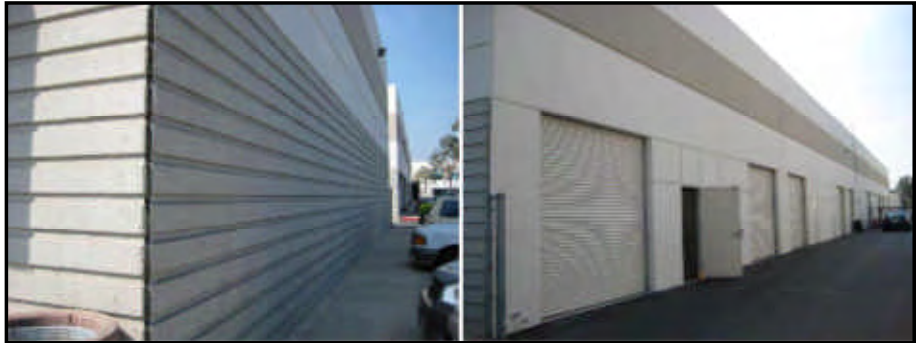
Concrete Tilt Up construction.
