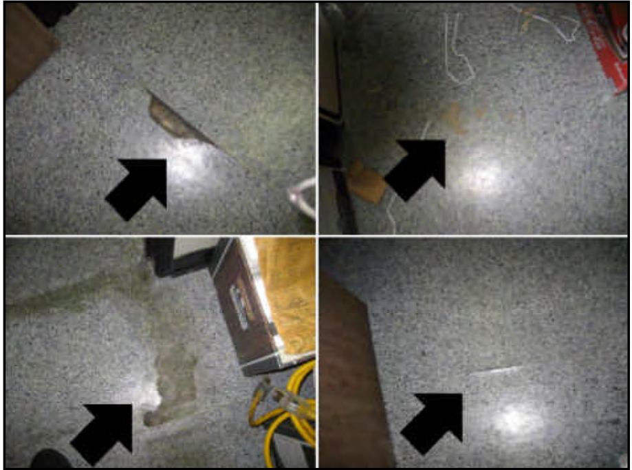
Pictures of the worn, damaged and aged linoleum.
