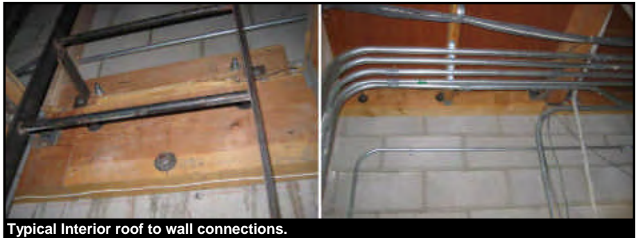
Typical Interior roof to wall connections.
