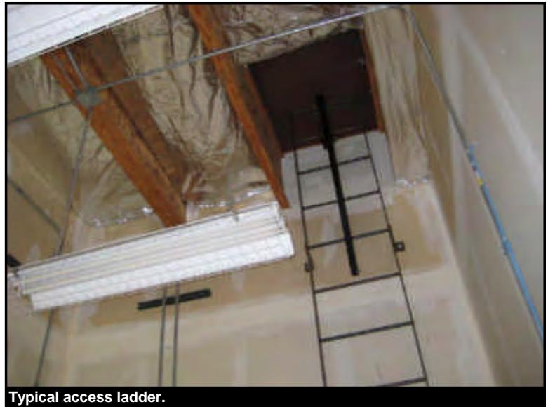
Typical access ladder.
