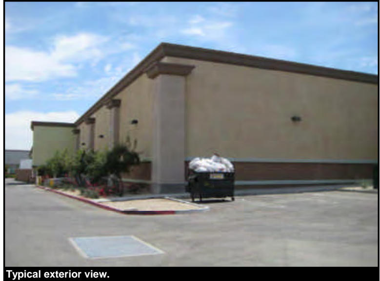
Typical exterior view.
