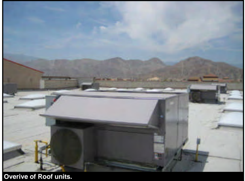
Overive of Roof units.
