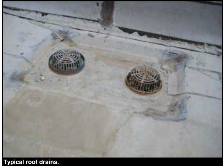
Typical roof drains.
