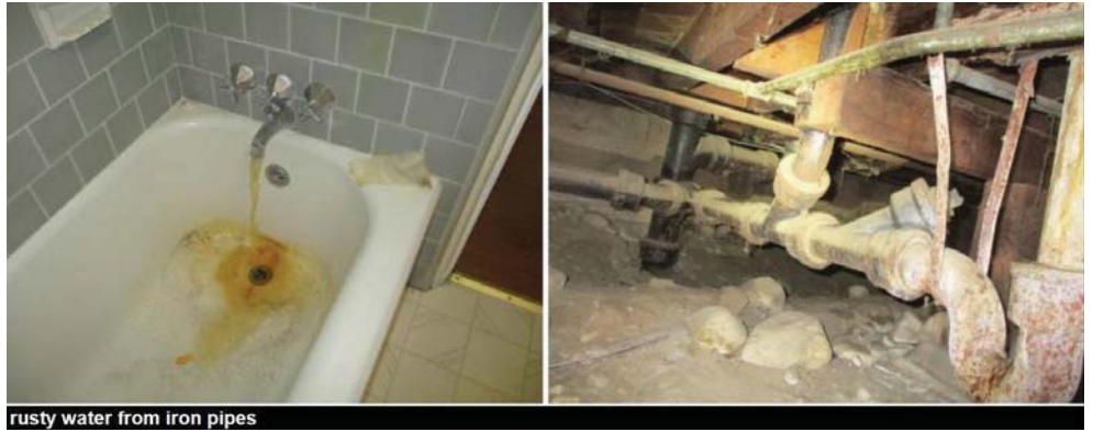
rusty water from iron pipes
