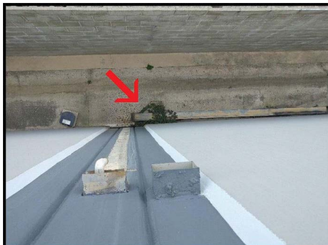
Disconnected downspout.
