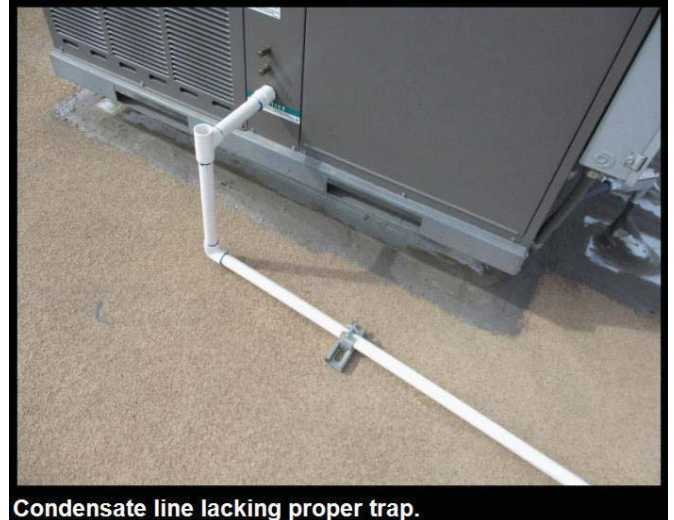
Condensate line lacking proper trap.
