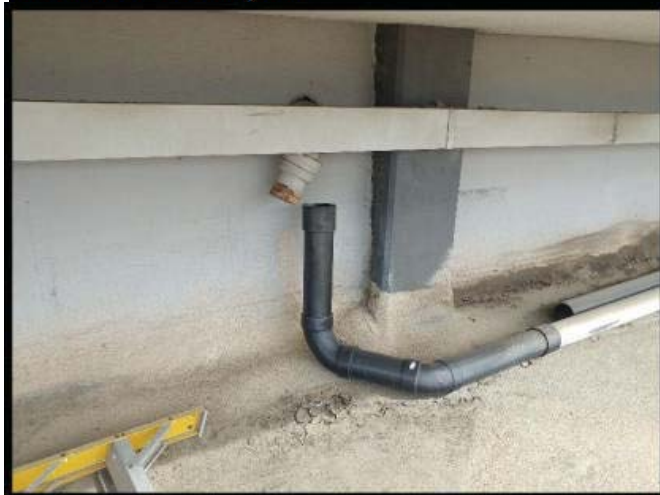
Disconnected downspout.
