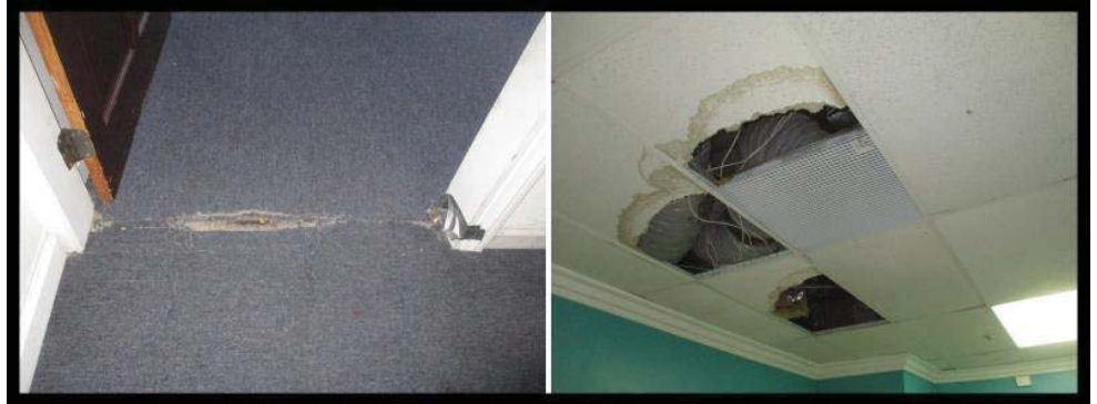
Unit 105 is vacant and has areas of missing light fixtures and worn flooring and wall and ceiling damage.
