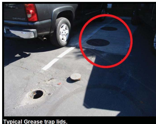
Typical Grease trap lids.
