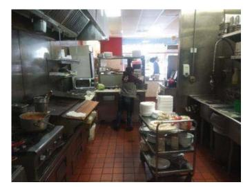
**Needs Attention:** There is a fire suppression system present in the kitchen. **Inspection of the fire** suppression system is beyond the scope of this general visual inspection however it is noted that the inspection tag was either missing or appears older. A detailed review is advised for health and safety.
