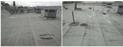
The roofing system has a Low Slope to it. This means that the slope of the roof appears to be no more than 2" of rise for every 12" of horizontal measurement.
