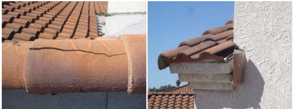
On the tile roof, there are areas of cracked/damaged tiles.
