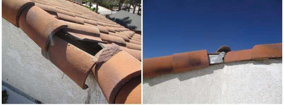
On the tile roof, there are areas of cracked/damaged tiles.
