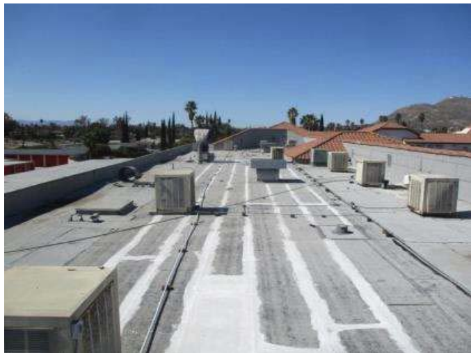
The roofing material on the low sloped roof is multi-layered roofing materials.
