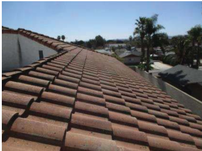
The roofing material on the sloped roof is made of concrete tile.
