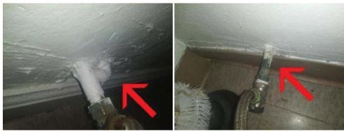
The interior piping that supplies the water throughout the building is made of copper where viewed.
