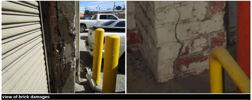
view of brick damages
