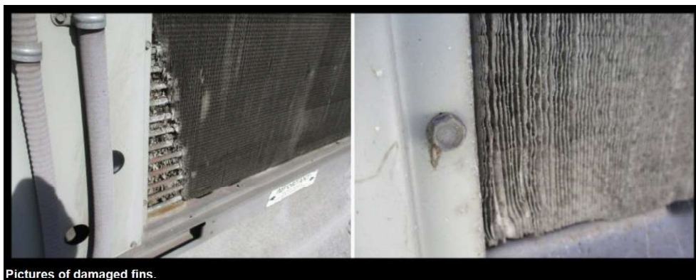
Pictures of damaged fins.
